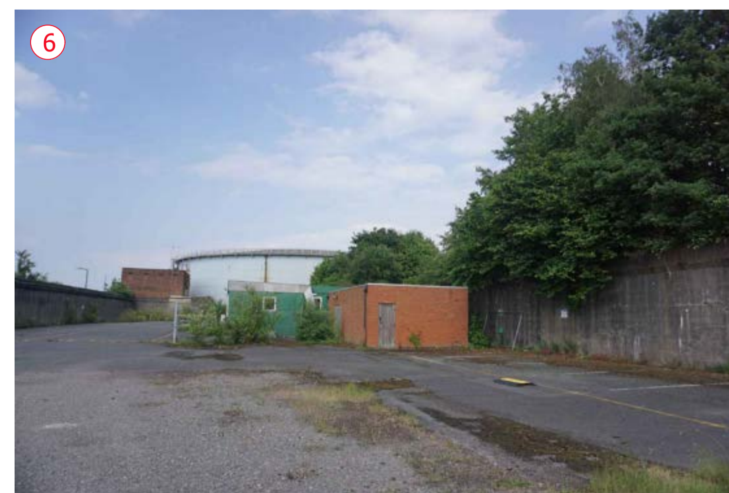
Outbuildings- to be demolished
