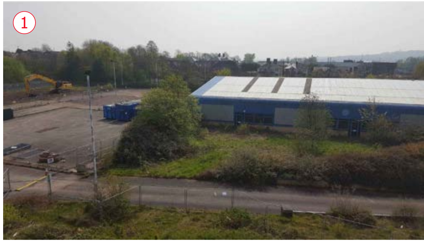
Existing office building. To be demolished
