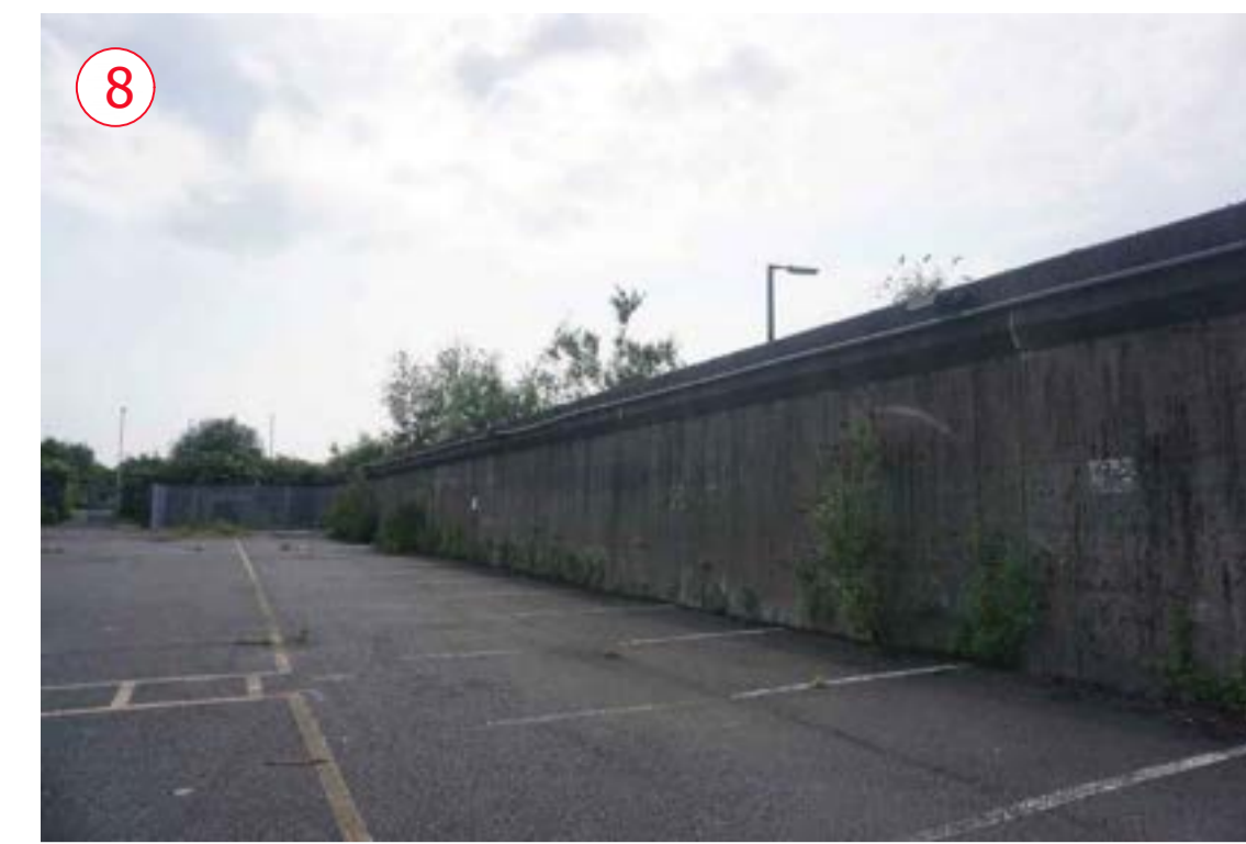
Concrete perimeter wall on north-west boundary
