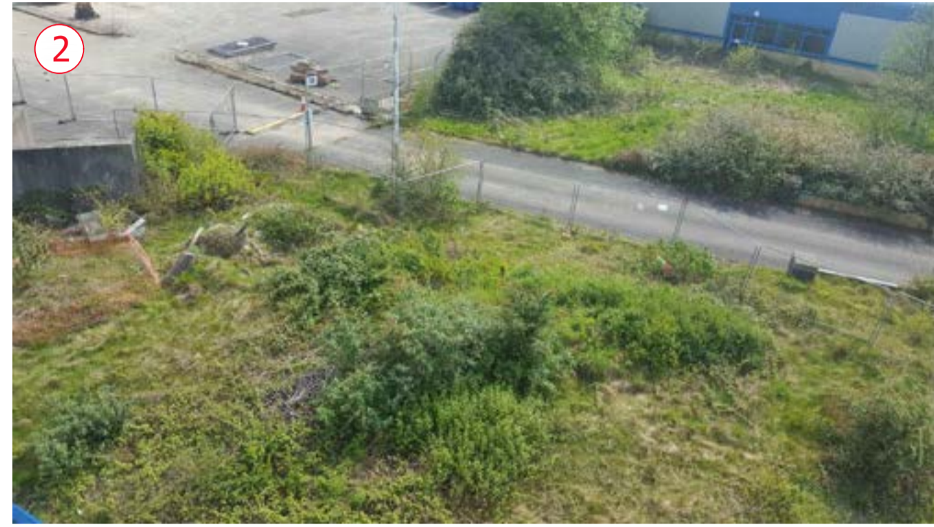
Internal access road along southern boundary
