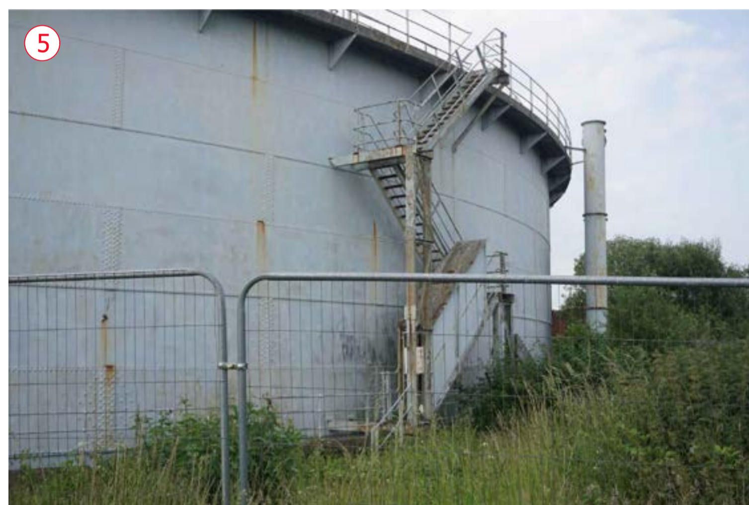
Gas holder 5 structure- since been demolished 2019.
